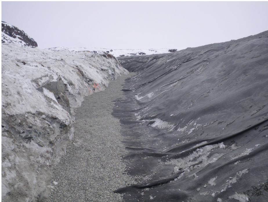
Photo 7: Diversion Berm – Bentonite plug placed in bottom of diversion berm. Photo looking east.
