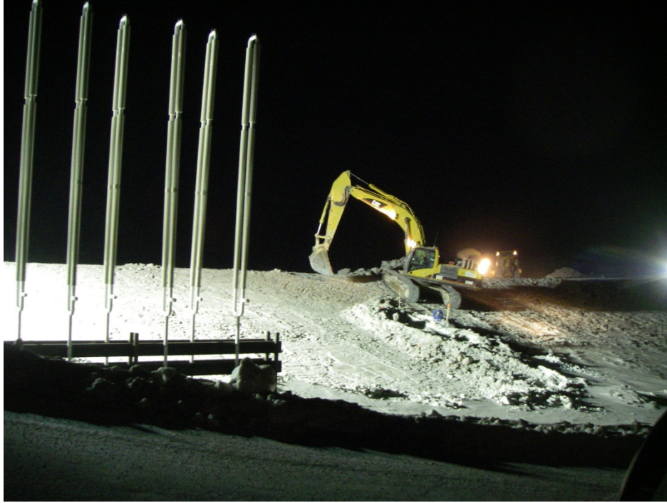
Photo 10: North Dam – excavator sloping and finishing the downstream face around Sta. 1+75. Photo taken from ice road, looking south
