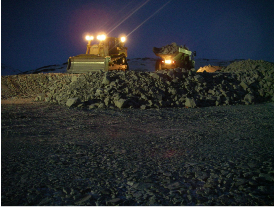
Photo 14: North Dam – progress photo of ROQ placement. Photo looking west from Sta. 0+80.
