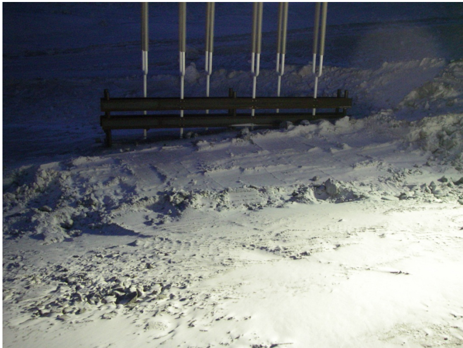
Photo 11: North Dam – snow cleared and crush surface levelled near the north thermosyphon radiators. Photo looking west.
