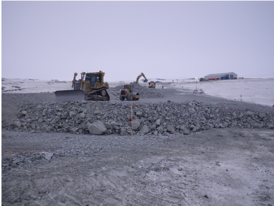
Photo 4: North Dam – View of progress on north dam. Dozer placing second lift of ROQ material over transition on upstream side of dam.
