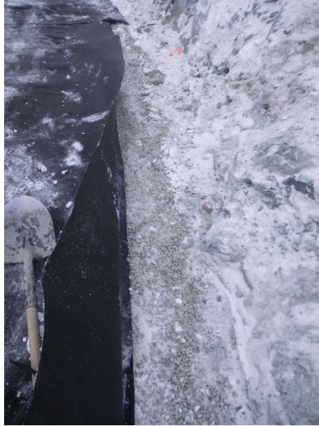
Photo 6: Diversion Berm – Closer view of bottom bentonite after snow cleaning.
